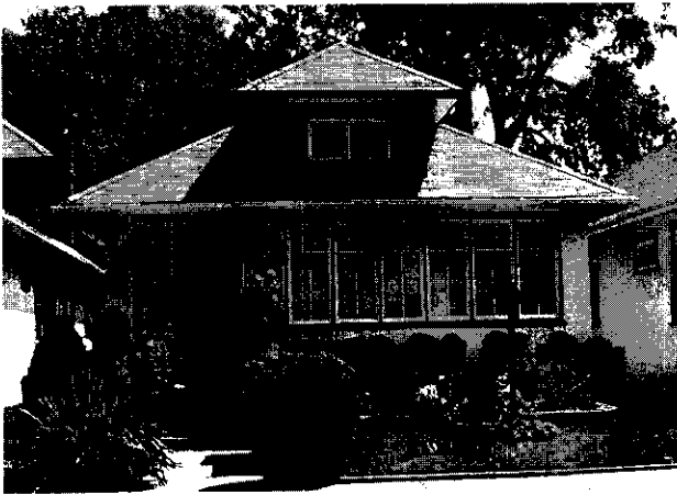
Figure 1: 7641 South Merrill Avenue
